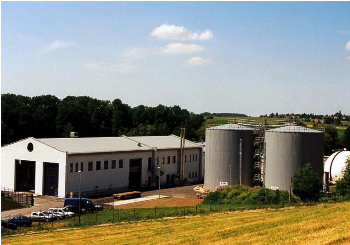
Fig. 1: Overall view of the Radeberg co-fermentation plant
