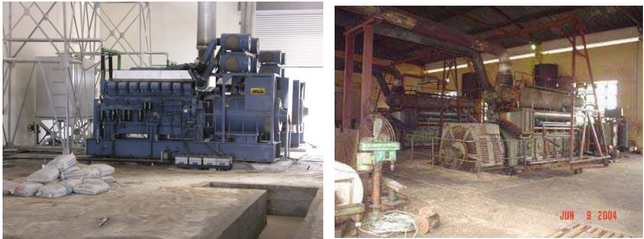
Figure 1: Power generation on Phu Quoc island: New power plant near the capital Duong Dong a- Diesel generators at the old generation site
