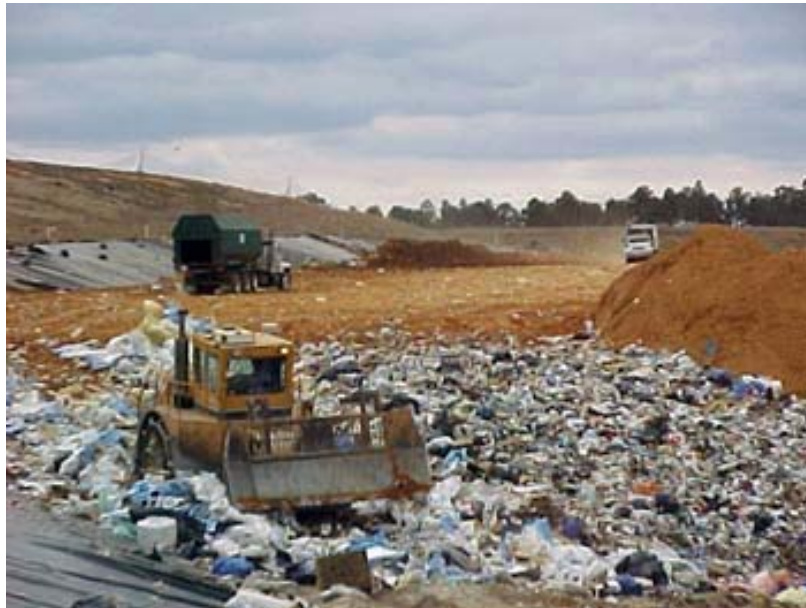
Figure 9: Landfill operation: liners are seen on the side of the area.
