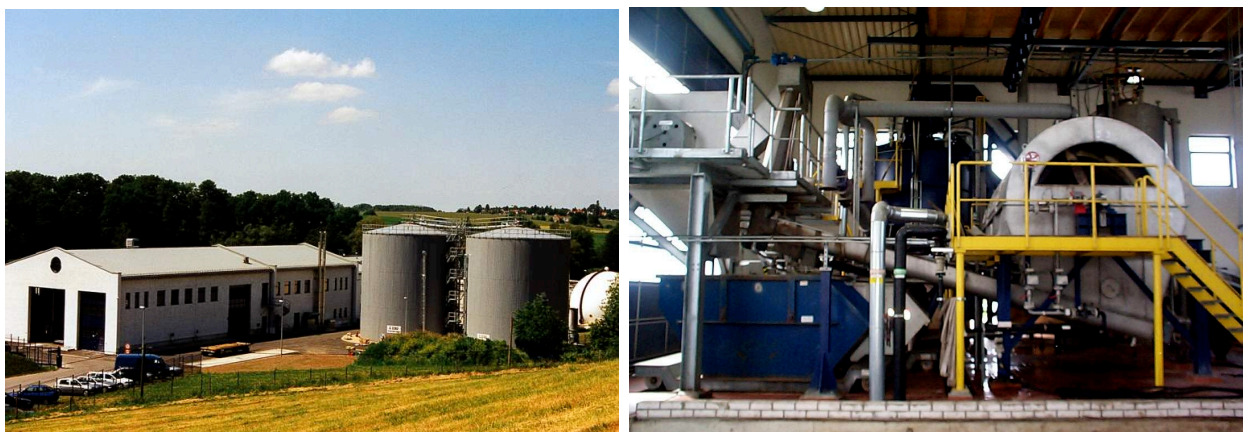
Abb. 2: Co-fermentation plant for solid, liquid and pasty waste, as well as for clarification sludge. Overview and mechanical treatment of solid co-substrates.
